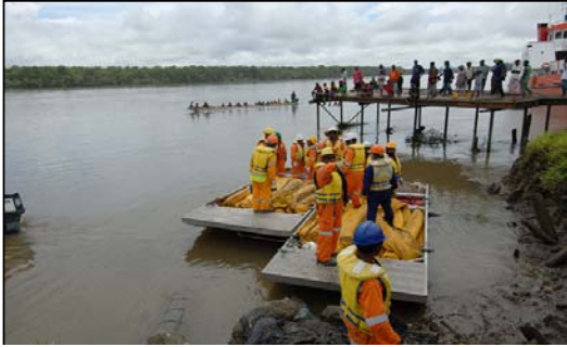
Fig 7.3 Preparation of booms at Kikori Jetty Source: Rockv Roe (OSL)
